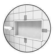
8. Add adhesive tape to hold the niche in place until the silicone has hardened.
